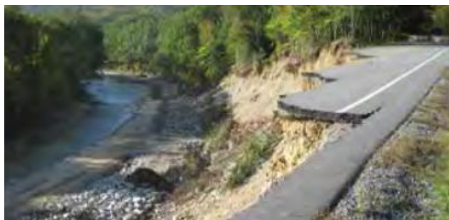
Tropical Storm Irene struck Vermont in August 2011 causing widespread damage across the State.
