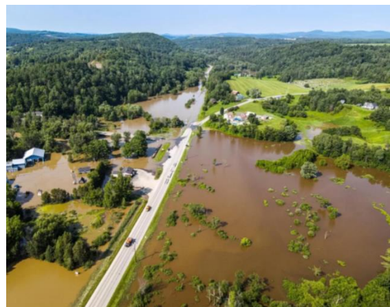
Significant rainfall in July 2023 resulted in flooding that caused significant damage to homes, businesses, and infrastructure across Vermont.
